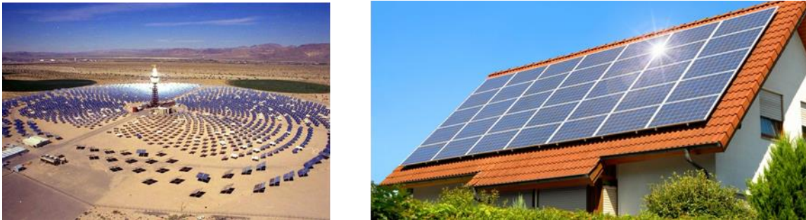
Figure 1.3: CSP system 4 (left) and PV system 5 (right).
